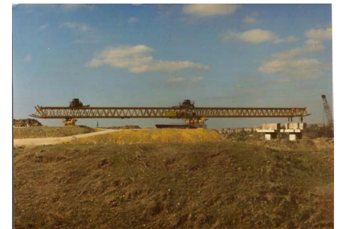
150 tons launching girder
