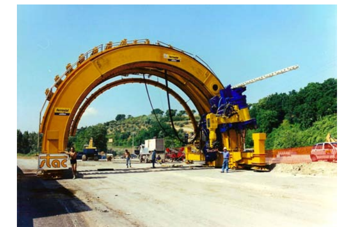
Multi-purpose equipment for tunnels enlargement without road traffic block
