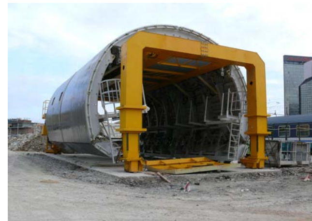
Formwork length: 10,00 mt Radius: 3,80 m
