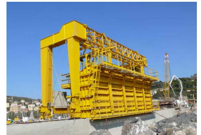
Breakwater wall self-mobile formwork
