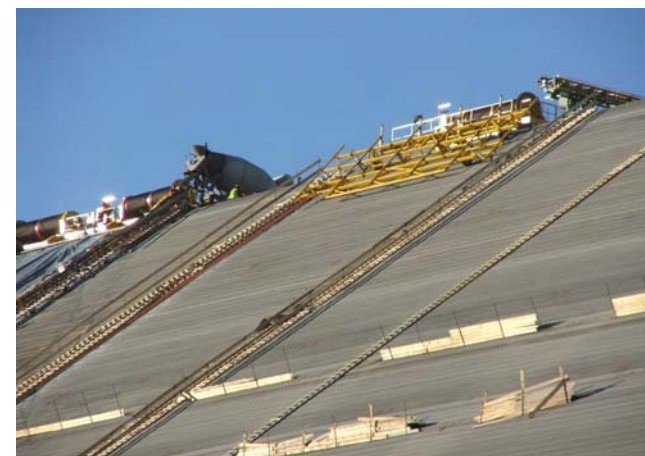
Dams face slab equipments
