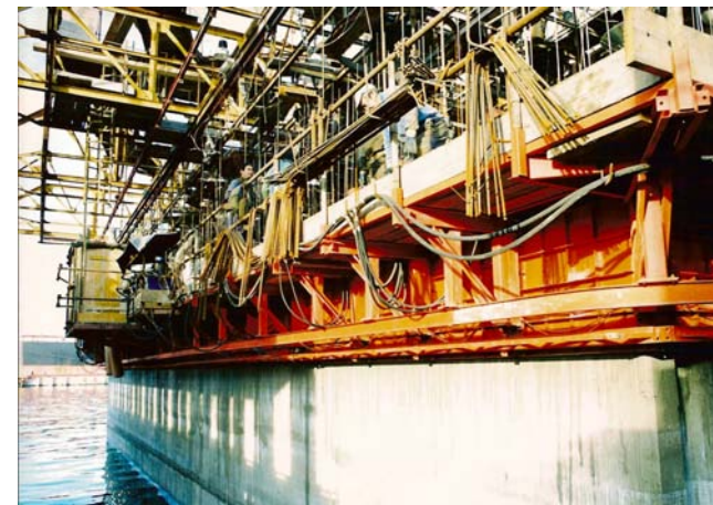
Concrete cellular tanks slip-forms
